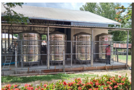
RFD room after completion
